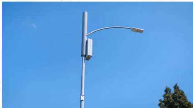
5G RF front end and antenna on light pole
