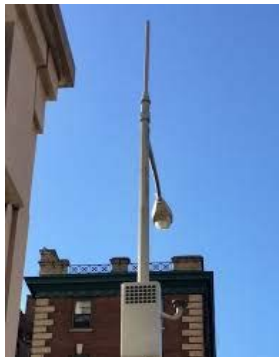
Sprint Massive MIMO and In-band backhaul @2.6 GHz
