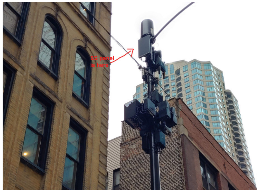
5G Base Station at 28 GHz on top of 4G LTE in Chicago on the Verizon Network [2].
