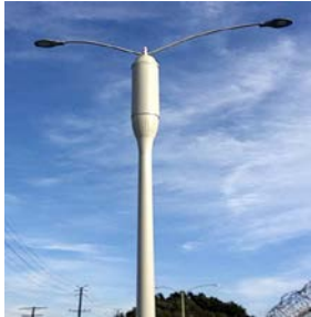
Streetlight small cells (CommScope).
