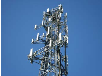
Cellular antennas on a lattice tower : low/mid band (Katherin)
