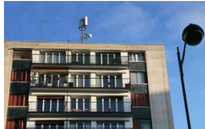
Cell sites on rooftops .
